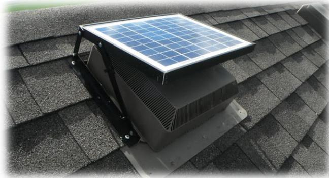
Mechanical Attic Ventilation via Solar Attic Fans
