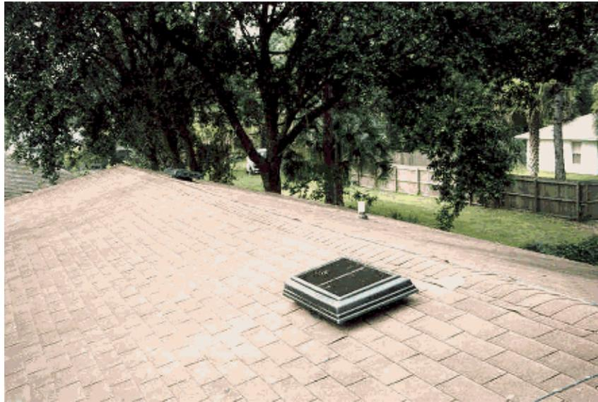
**Figure 2.** Photo of PV ventilators.
